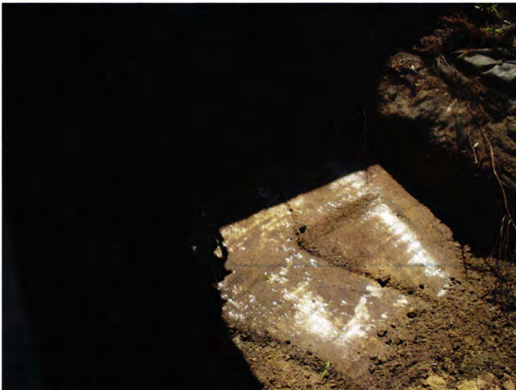
Picture 2: UST 331Ash excavation in progress.
